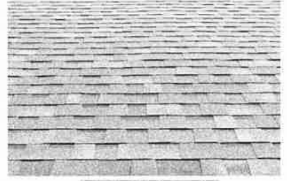
Asphalt shingles for the roof and side walls, Ref image below:
