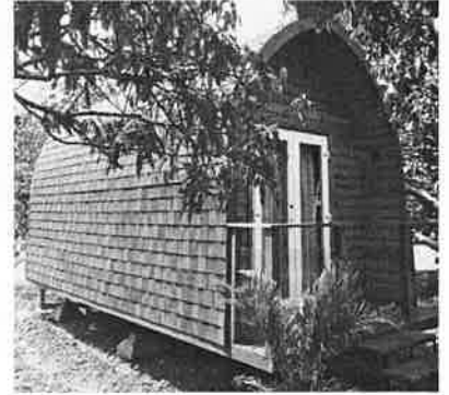
Asphalt shingles for the roof and side walls, Ref image below:
